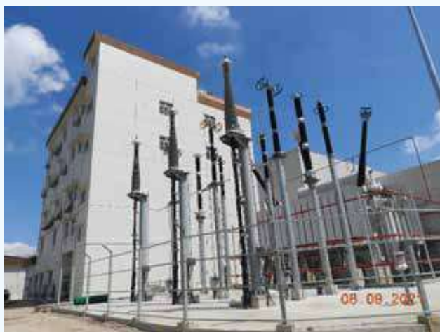
Generator Step-up Transformer
